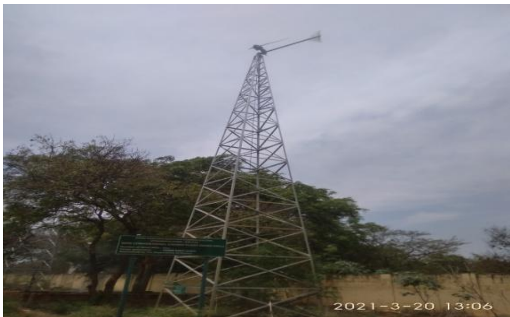
Fig.11: Lattice tower Horizontal axis Wind turbine
