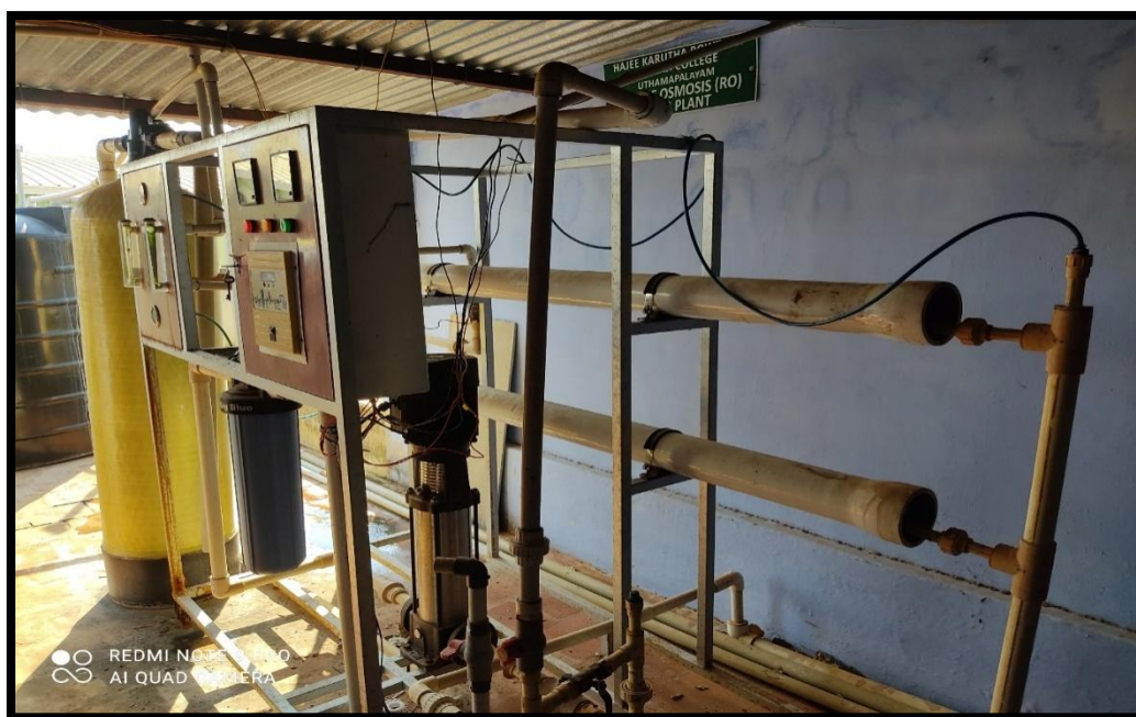
Fig.2: Reverse Osmosis (RO) Plant
