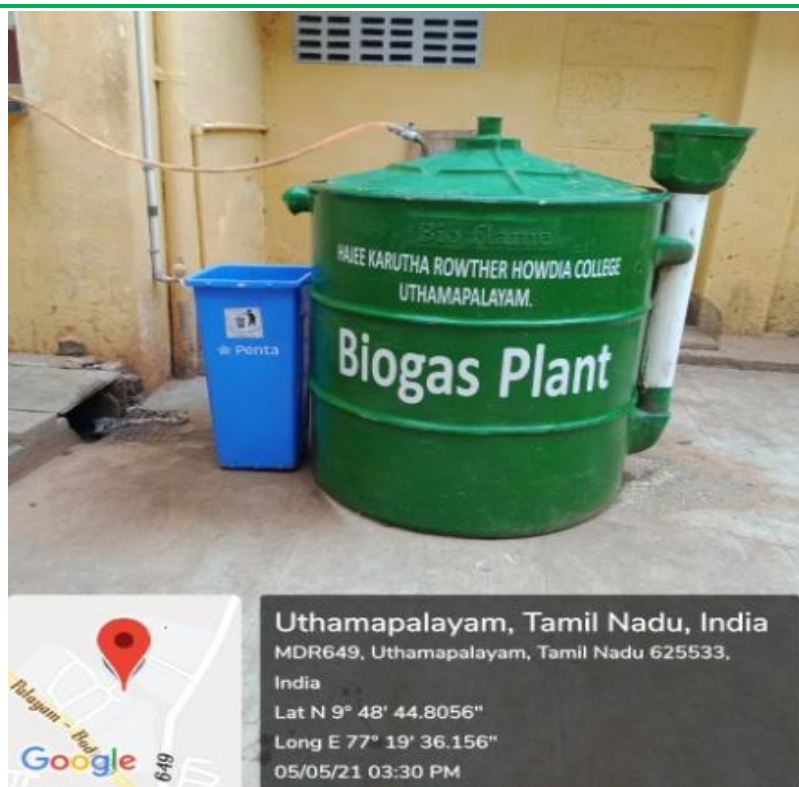
Fig.6: Floating type Biogas plant
